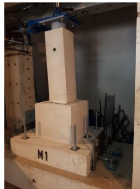
Figure 19. Start damage at RC column
