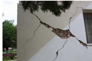
Figure 3B. Close view from exterior wall
